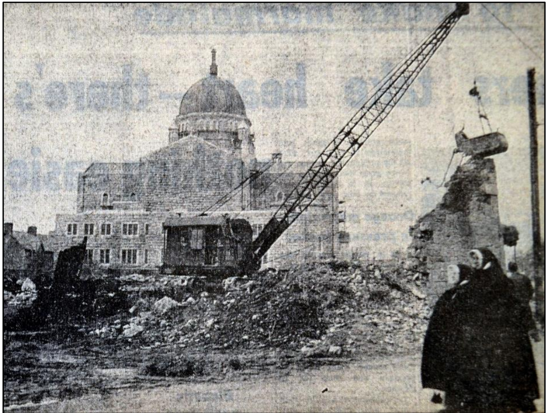
Fig. 7. The demolition of the boundary wall of the former execution yard at Galway jail. From the Irish Press , 12 Jan. 1965.
