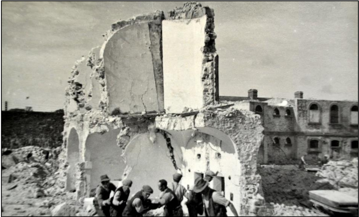
Fig. 3. Men demolishing Galway jail during the ‘Emergency’ years, c. 1941–43. From Galway Diocesan Archives, Bishop Browne papers, B/6/8.
