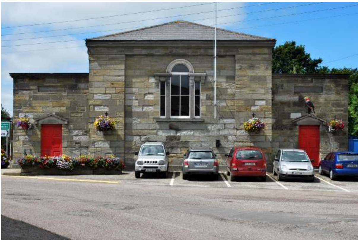
Fig. 1. Clonakilty courthouse and bridewell, main façade. Author’s photograph, 2013.
