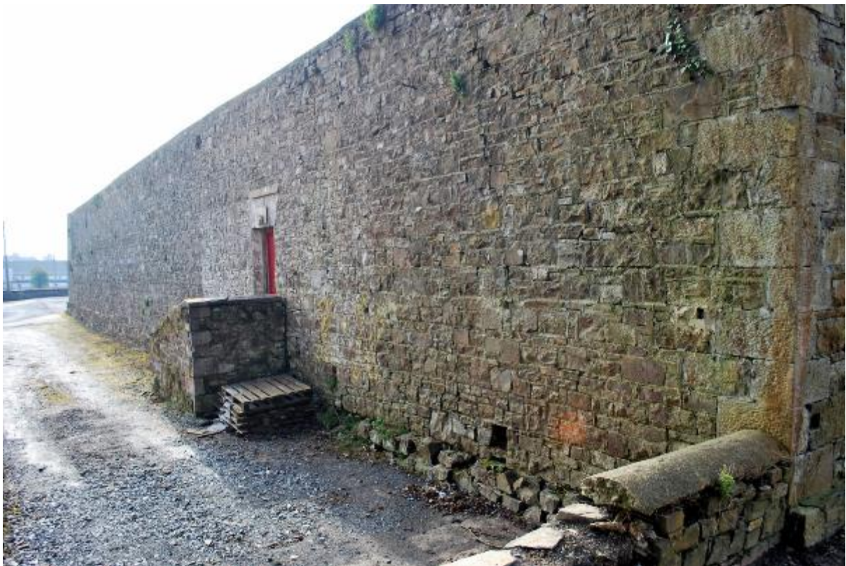
Fig. 7. Kanturk bridewell, outer perimeter wall, from the north-west. Author's photograph, 2013.
