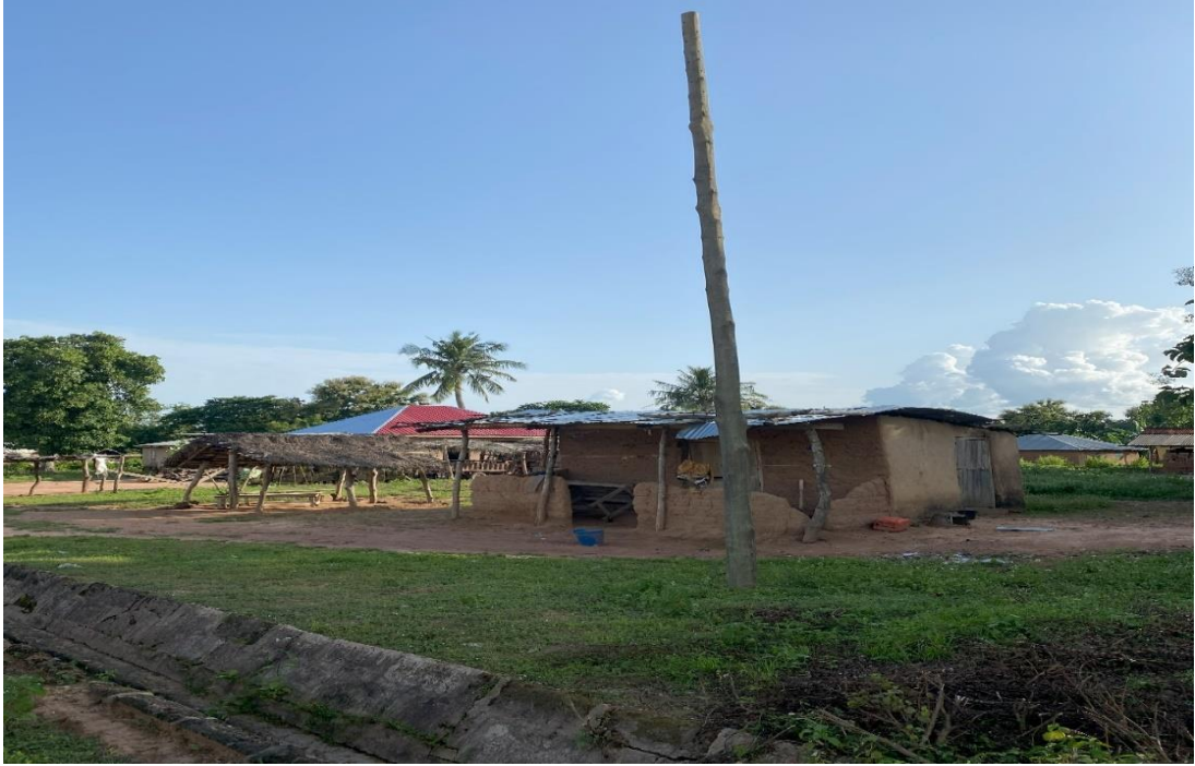
Image 2: A rural community with an erected electric pole waiting to be connected to the national grid
