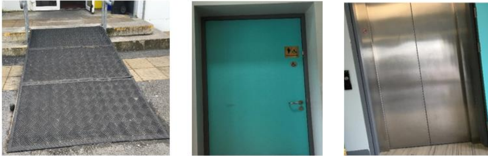
Figure 5.3. Wheelchair Accessible Facilities in School
