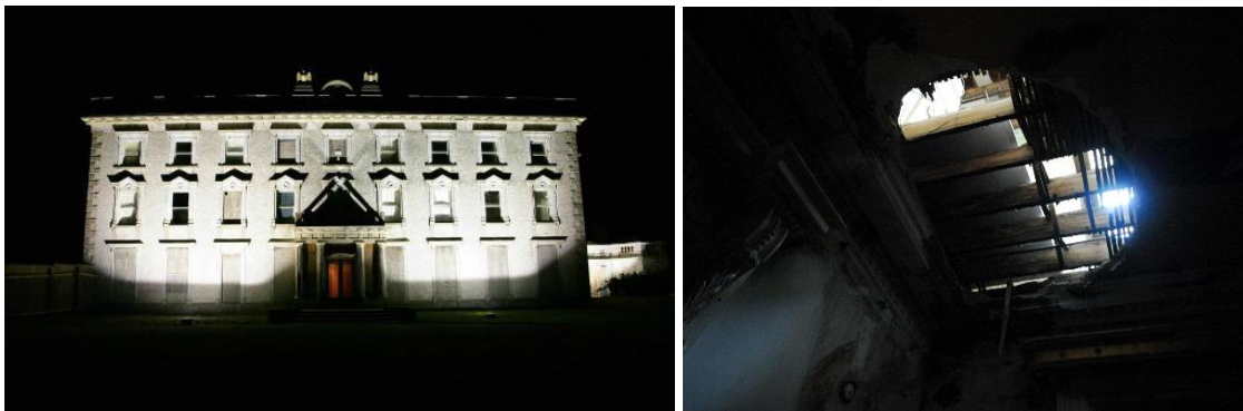
Figs. 60-61: Loftus Hall (c. 1760): (From left to right): Façade; Hole in roof.
