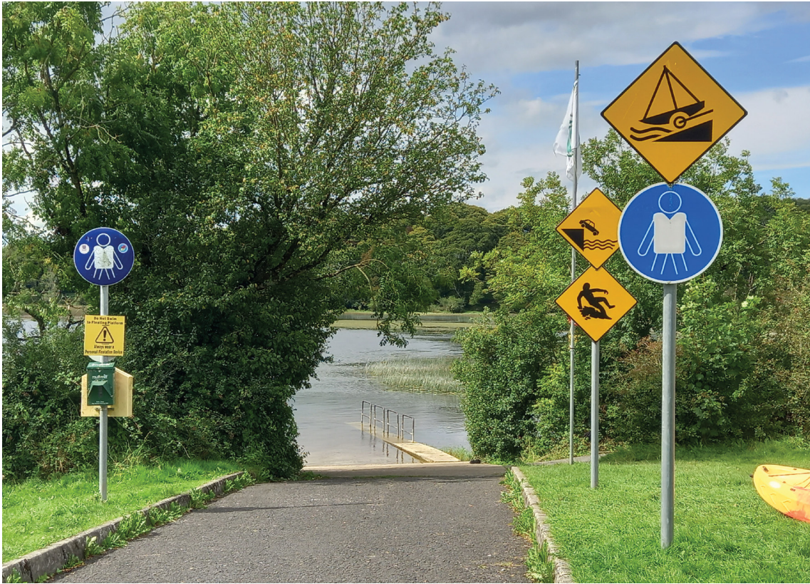
Figure 18.2 Public access boat slipway, Ballyallia Lake (Clare)
